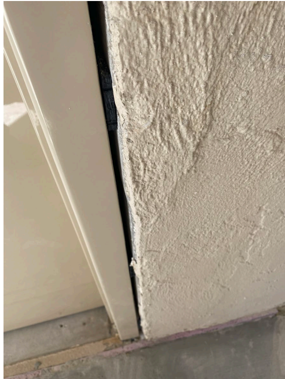
Picture 6: Typical use of shims
