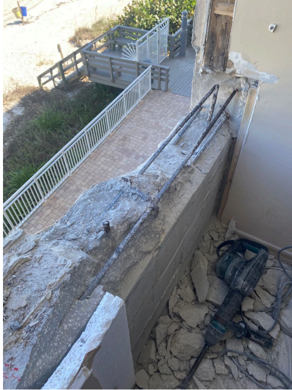
Picture 5: Unit 208 in-progress window sill repair
