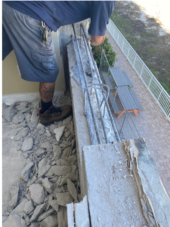
Picture 4: Unit 209 window sill repair
