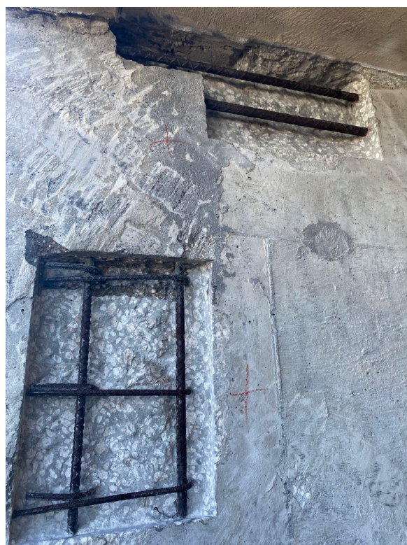
Picture 2: Approved excavation
