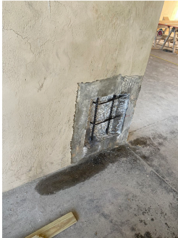
Picture 3: Approved excavation
