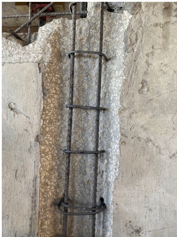
Picture 1: Approved excavation
